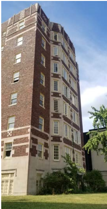
Fig.3 East and partial south elevations. Photo: IHPC Staff, 2019
