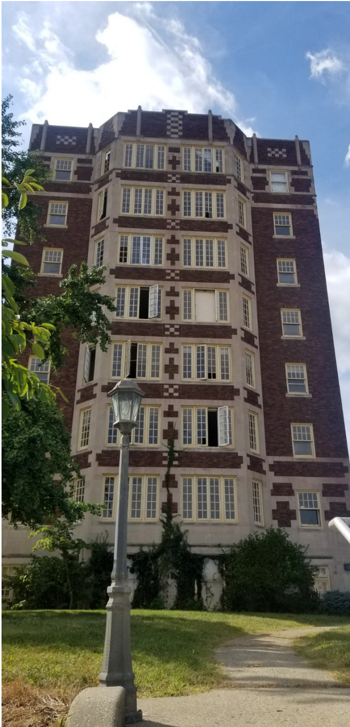
Fig.1 East elevation. Photo: IHPC Staff, 2019
